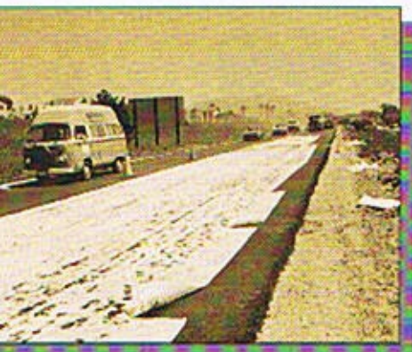
Dual-sided heatbonded fabrics are thin and stiff and have a tendency to curl up when installed by hand.
