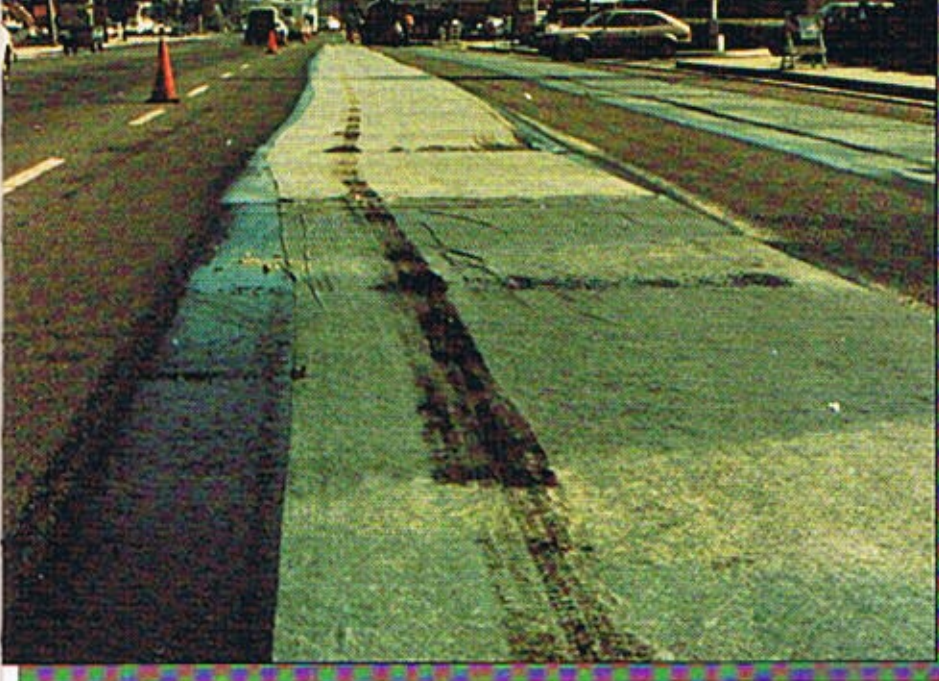
Delamination and slippage can occur if the fabric's heat-bonded side is not placed up.
