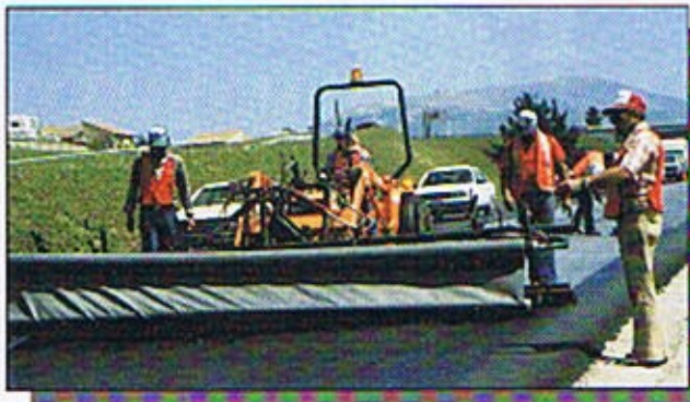
Sometimes wrinkles are rolled into the roll at the factory, but mechanized equipment can remove many wrinkles prior to placement.
