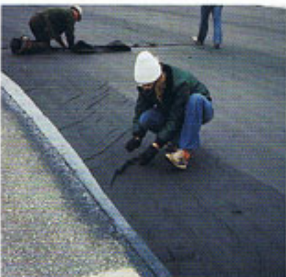
Figure E: Wrinkles are a fact of installation. But, minimizing them and proper slitting assure a quality job.
