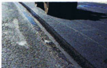
Figure F: Fabric overlaps from adjoining lanes should be six inches. When overlaying adjoining lanes, AC should be held back to ensure lap length.
