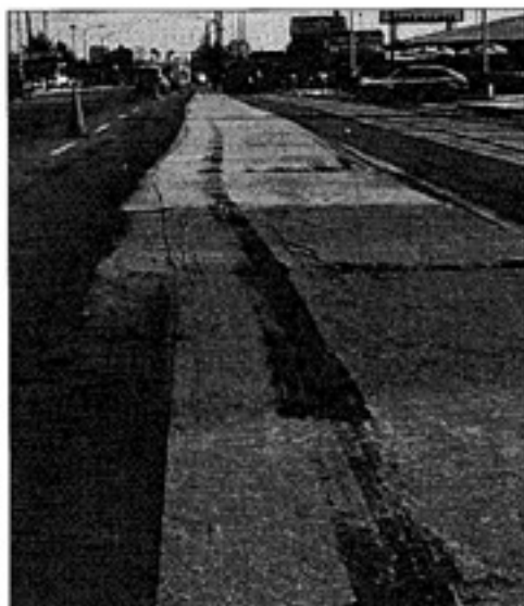
This heat bonded needlepunched fabric was placed upside down.
