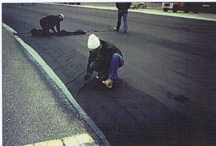
Manually rolling and brooming the fabric by hand can be a time consuming and slow process and requires additional workers.
