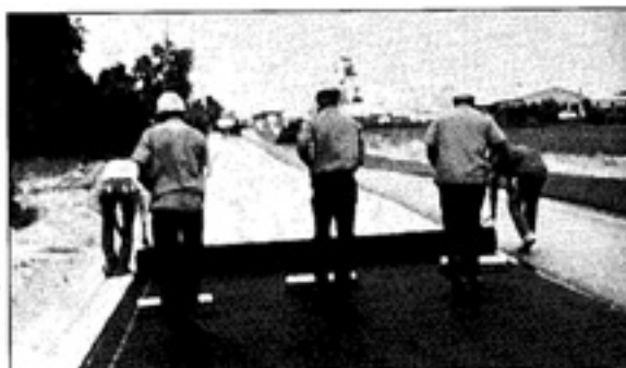
After wrinkles are cut, all overlapped wrinkles and all overlaps in the fabric should have an additional tack coat applied.
